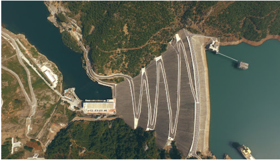
Figure 4. Fierza HPP and Power Station
