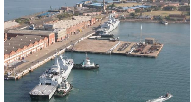
Expanded autonomous and intermodal naval facilities to cater for future ambitions of national and allied navies
